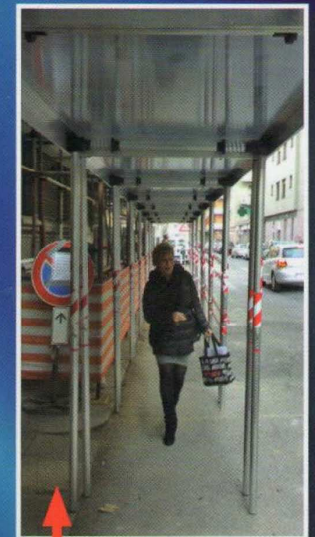
PROTECTED CORRIDOR WITH FIXED OR MOBILE SCAFFOLDS
